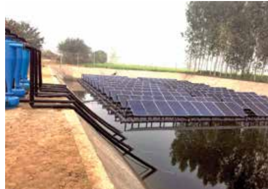
Submersible pump testing
