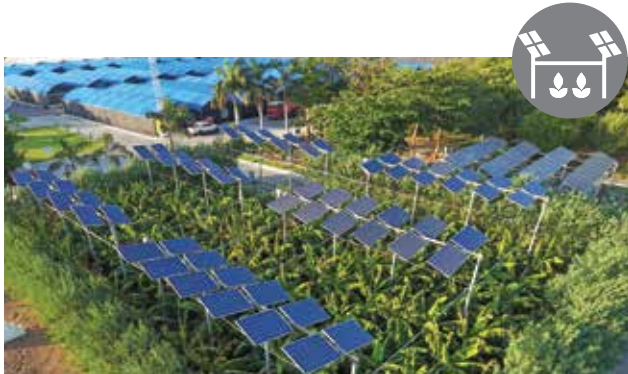
Solar AgroVoltaic Plant
