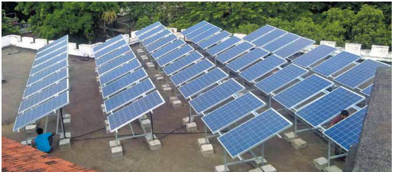
Roof Top Structure
