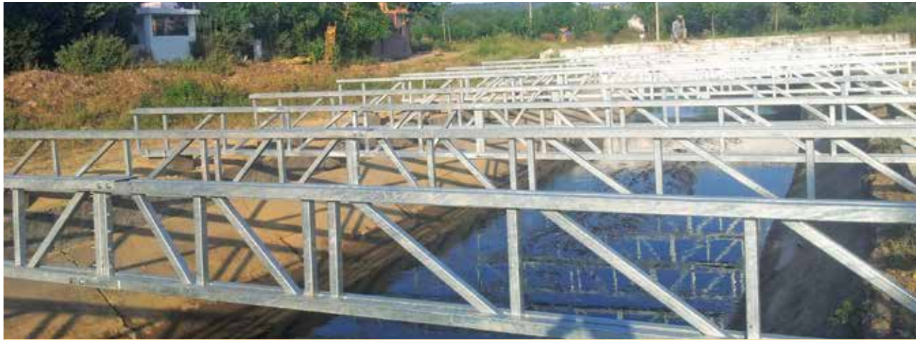
Canal Top Structure
