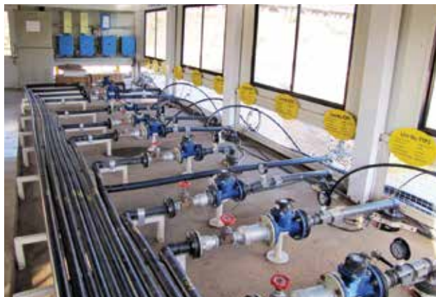
Pump testing setup
