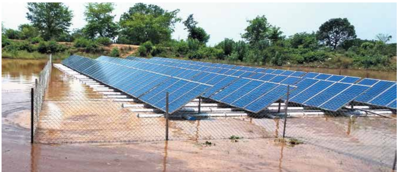
Jain Tarang (Floating) Platform in reservoir
