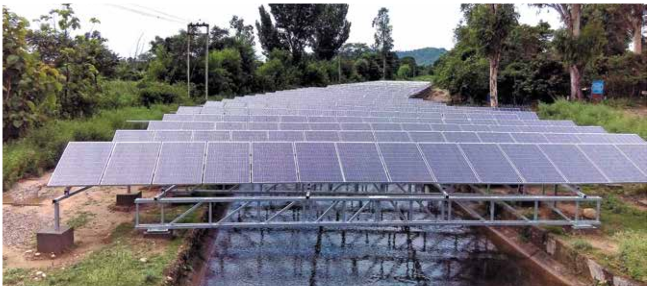
Canal Top Structure
