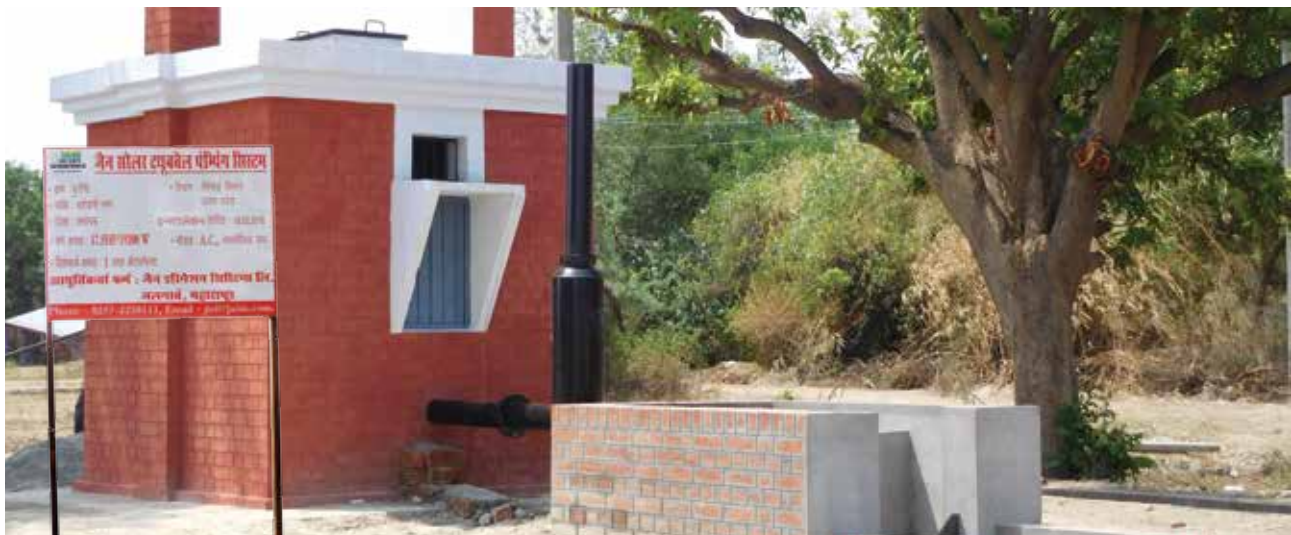
Community Tube Well Pump House
