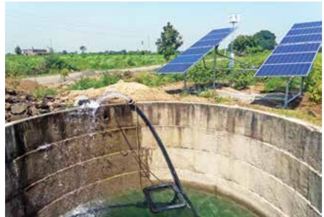
Jain Tarang (Floating) Platform in Open Well
