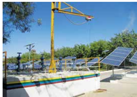
Surface pump testing
